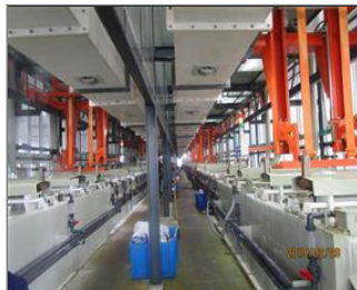
Photo of the inside of the main production hall Electroplating workshop.JPG
